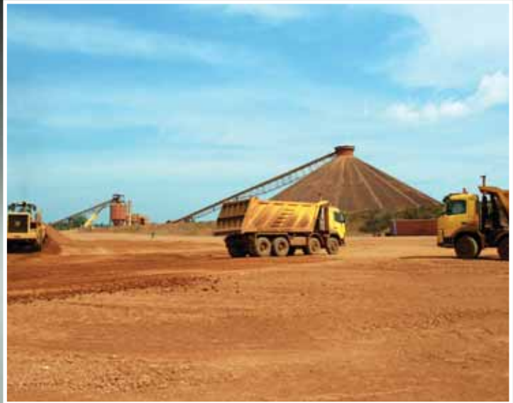
Bauxite dryer and storage dome, SML Bauxite mine
