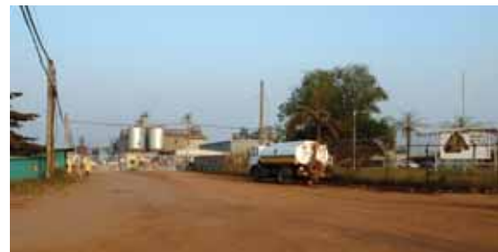
Water bowser carrying out road surface dust suppression SRL dry plant
