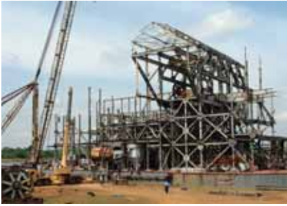
Dredge D2 under construction, Sierra Rutile mine
